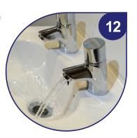
Check the outlet at the tap and note the now reduced flow rate.
