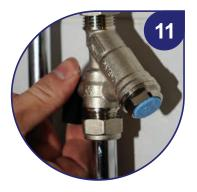
Tighten the cap, turn on and check for leaks.
