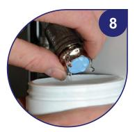
Allow the valve to drain and then flush through any installation debris.
