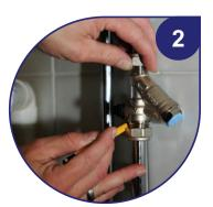
Isolate and drain the supply then mark the area of pipe that needs to be removed. (52mm)
