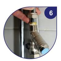
Having measured and cut the correct amount of tube, install the nut and olive for the outlet
