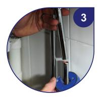
Making sure the water supply is off, use a suitable cutting tool to remove the pipe taking care to leave room for installation and future servicing.
