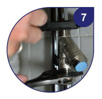
Isolate and turn water on to check the inlet connection for leaks. Reinstate water supply and check the top connection for leaks. Isolate again and remove the plug over a suitable container.
