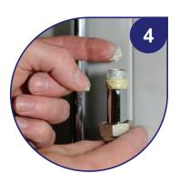
Fit the nut and olive over the now open end of the tube using a suitable sealing compound around the olive.
