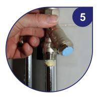
Insert the BOSS™ 282 CF Calflow® Plus body into the supply pipe taking care to make sure the tube reaches the "stop" points in the valve body. Check the direction of flow.
