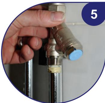
5 Insert the BOSS™ 282 CF Calflow® Plus body into the supply pipe taking care to make sure the tube reaches the "stop" points in the valve body. Check the direction of flow.
