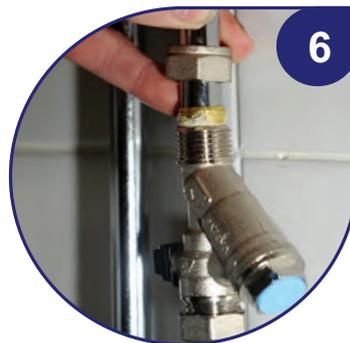
6 Having measured and cut the correct amount of tube, install the nut and olive for the outlet
