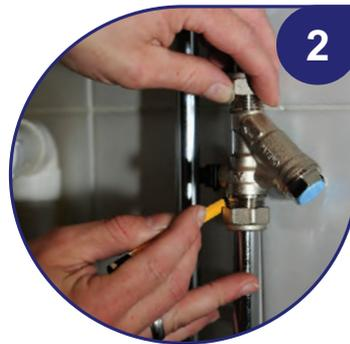
2 Isolate and drain the supply then mark the area of pipe that needs to be removed. (52mm)
