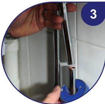
3 Making sure the water supply is off, use a suitable cutting tool to remove the pipe taking care to leave room for installation and future servicing.
