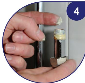
4 Fit the nut and olive over the now open end of the tube using a suitable sealing compound around the olive.
